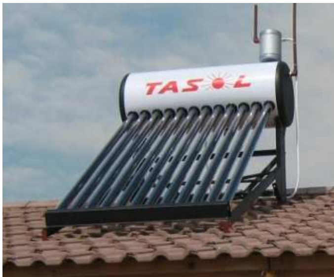
Figure 1. Low pressure vacuum tube collector SWH system
